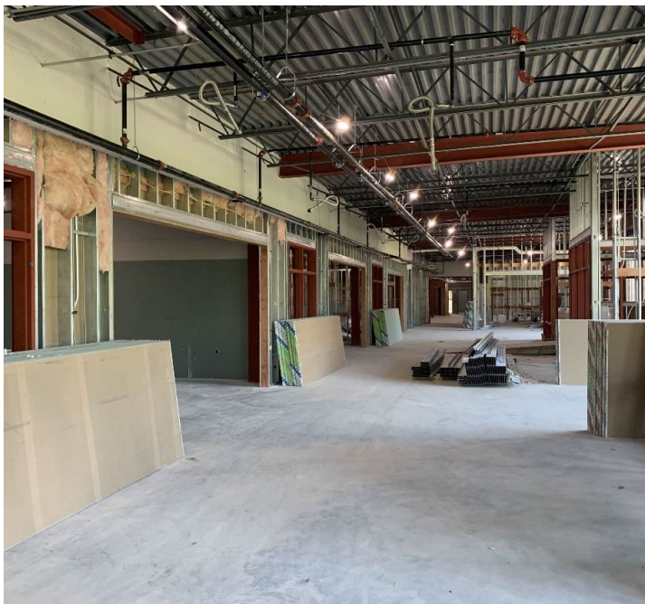
Metal stud framing and sprinkler piping installation is underway.
