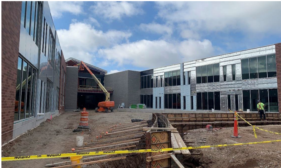
Concrete seat walls are being formed and poured.
