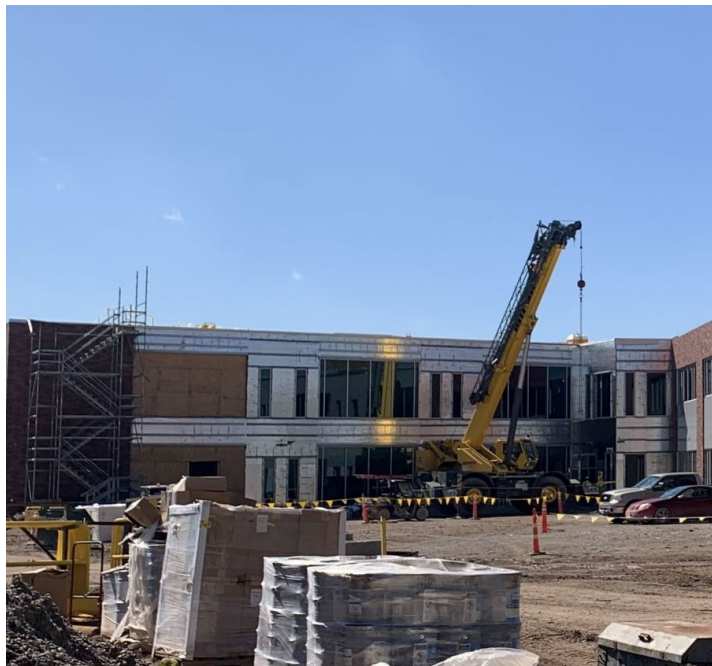
Board insulation has been installed.
